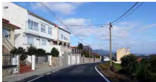
Ribeira (A Coruña). Two-way road section with horizontal signs only on the sides
