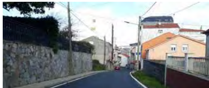
Note the different treatment for sidewalks on road sides. Is it adequate or inadequate? This type of decisions must be justified in the project
